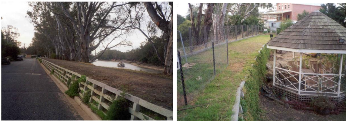
Figure 8 Crib Wall levee constructions
