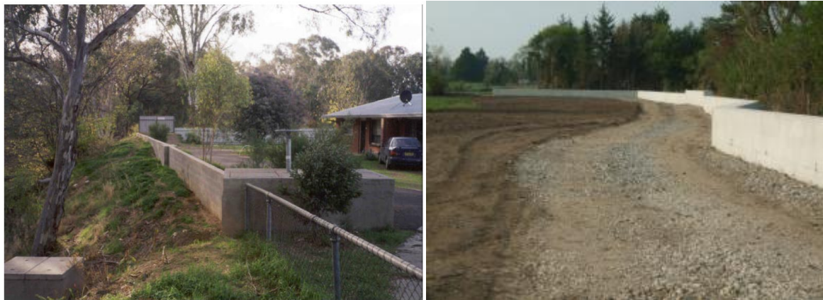
Figure 9 Concrete Retaining Wall Levee Constructions
